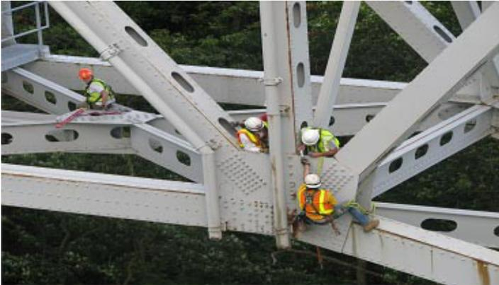
Current inspection techniques on a single plate can take over 30 minutes. However, the Pocket UT™ System and R-scan can inspect the same area in less than 5 minutes, taking readings every .050", and saving all the data to produce a graphic image of the area with no couplant required.
